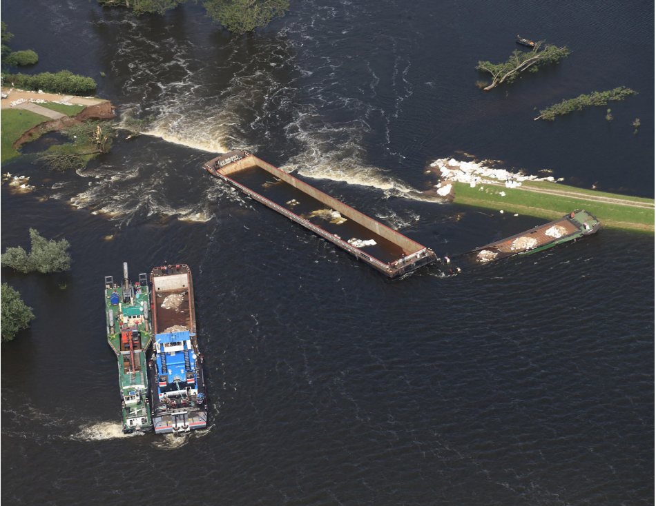
Figure 3: A levee breach in Fischbeck led to a risky manoeuvre to sink three barges in order to plug the gap.
